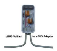
The company that supplies the Modbus system will then continue the eBUS connection from this junction box to enable sub-distribution with the Modbus Gateway (this junction box also serves to separate the eBUS connection for servicing).
